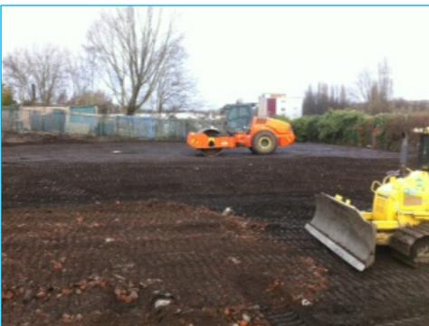
The geotechnical design proposal was to remove 3m of made ground, (63,000m<sup>3</sup>) removal and process of all relic foundations, place a load transfer platform (LTP) at 0.3m of 6F2 with geogrids and reinforcing membrane, then re-engineer the site with fill to finished level (minus construction depth) in class 1 graded, engineered and tested general fill to the Specification to Highways Works (SHW) Series 600.
