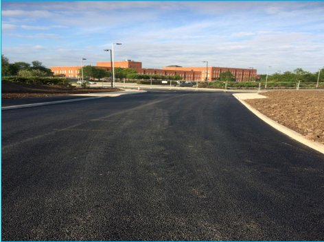
Access Road Works
