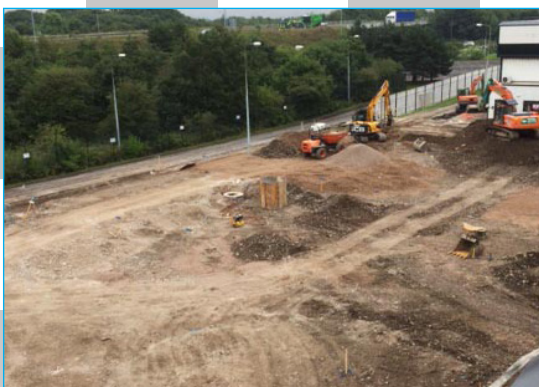
Earthworks and Drainage Phase
