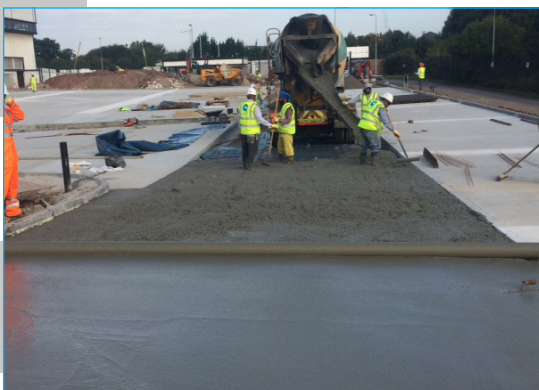
Concrete Road Construction
